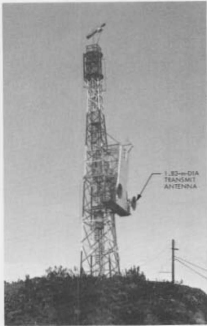
Fig. 5. DSS 13 collimation tower and 1.83-m (6-ft) diameter transmit antenna. The S-band feed shown in photograph was replaced by an X-band feed
