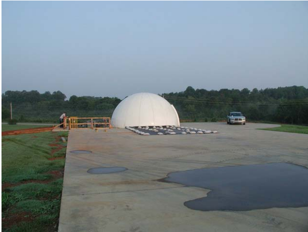
Figure 1. Carlex Glass Vehicle Antenna Test Site
